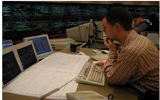
Figure 1. Time-distance graphs on paper are a main tool in today's control of train traffic.
